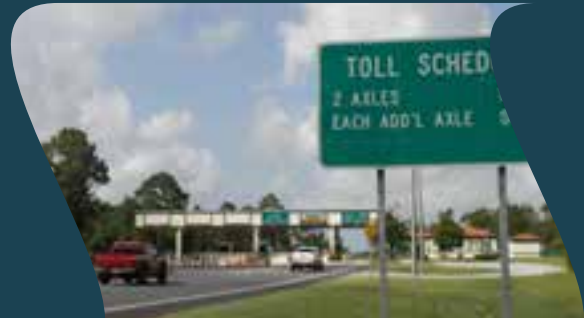
GARCON POINT BRIDGE
