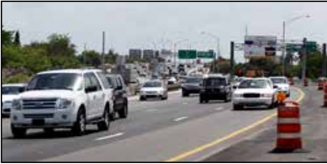
95 Express Phase II construction.
