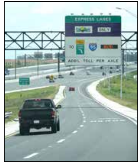
Eastbound entrance ramp onto 595 Express.
