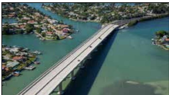
Pinellas Bayway System replacement bridge on SR 682
