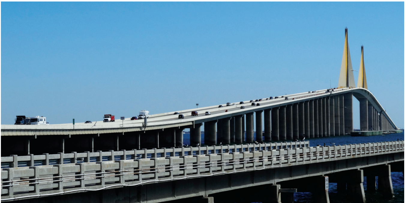
Sunshine Skyway Bridge
