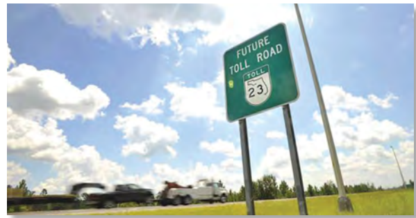
The First Coast Expressway is currently under construction in the Jacksonville area.
