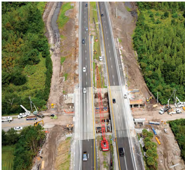
Veterans Expressway widening
