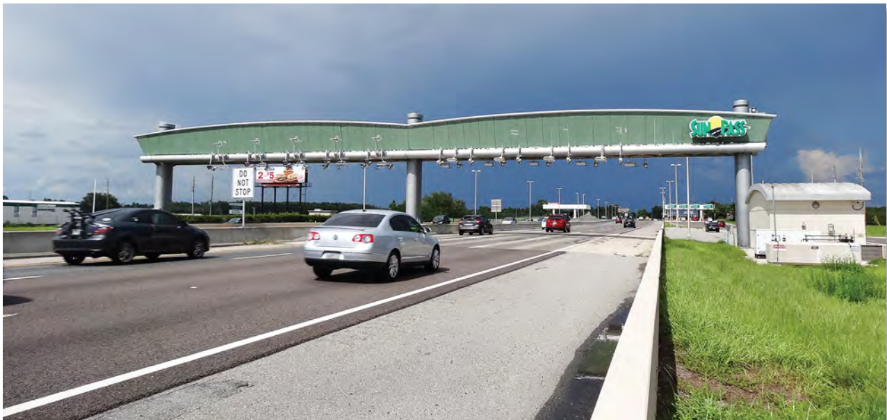
All-Electronic Tolling is a highly efficient means of collecting tolls.
