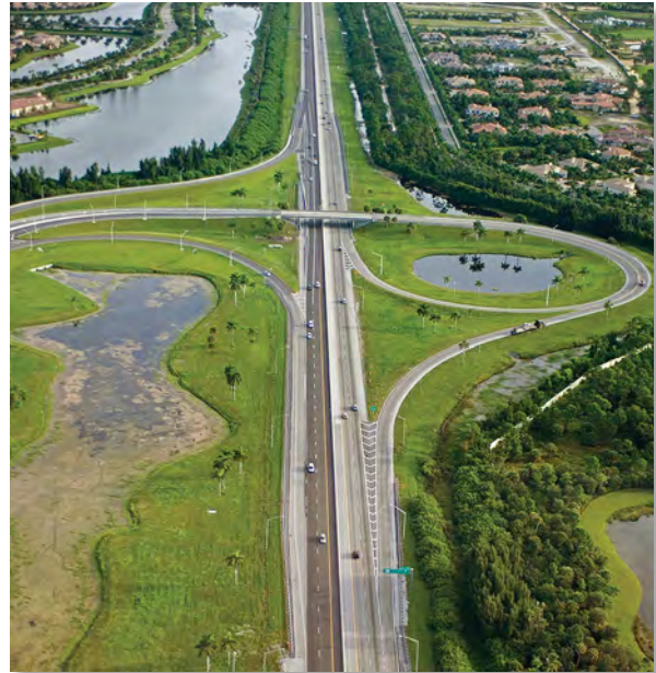
Palm Beach County resurfacing
