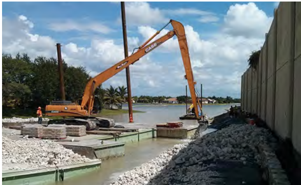
Sawgrass canal revetment
