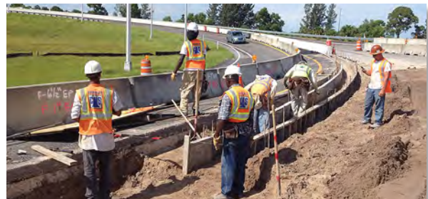
Milepost 116 Indiantown Road construction
