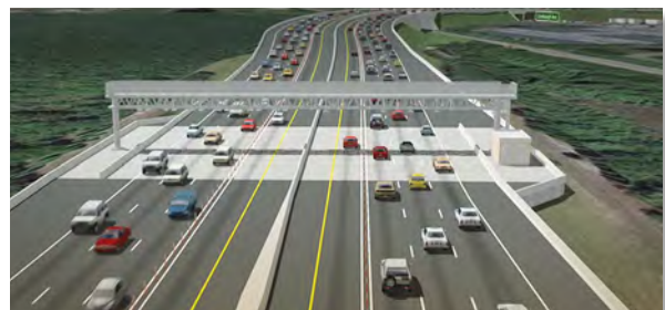
Rendering of future AET gantry north of previous Anderson toll plaza on the Veterans Expressway
