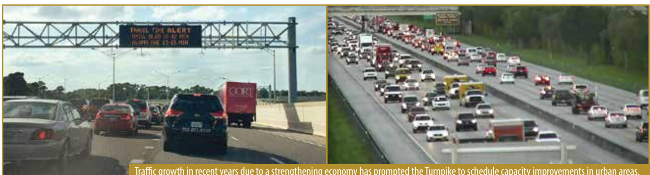
Traffic growth in recent years due to a strengthening economy has prompted the Turnpike to schedule capacity improvements in urban areas.
