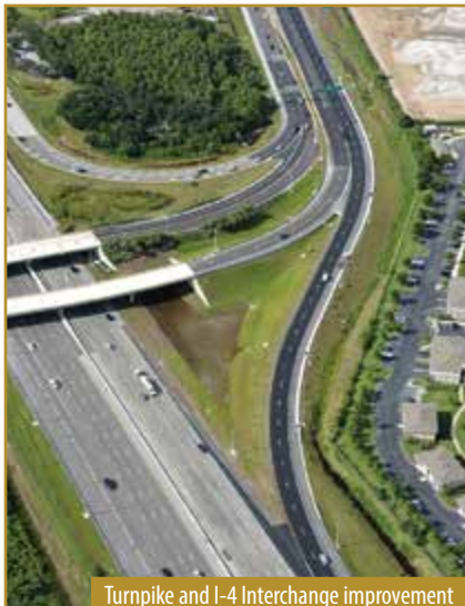
Turnpike and I-4 Interchange improvement
