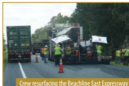
Crew resurfacing the Beachline East Expressway
