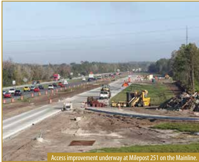
Access improvement underway at Milepost 251 on the Mainline.
