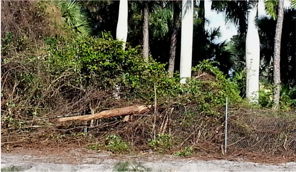
Figure 11 – Condition of Existing Fence
