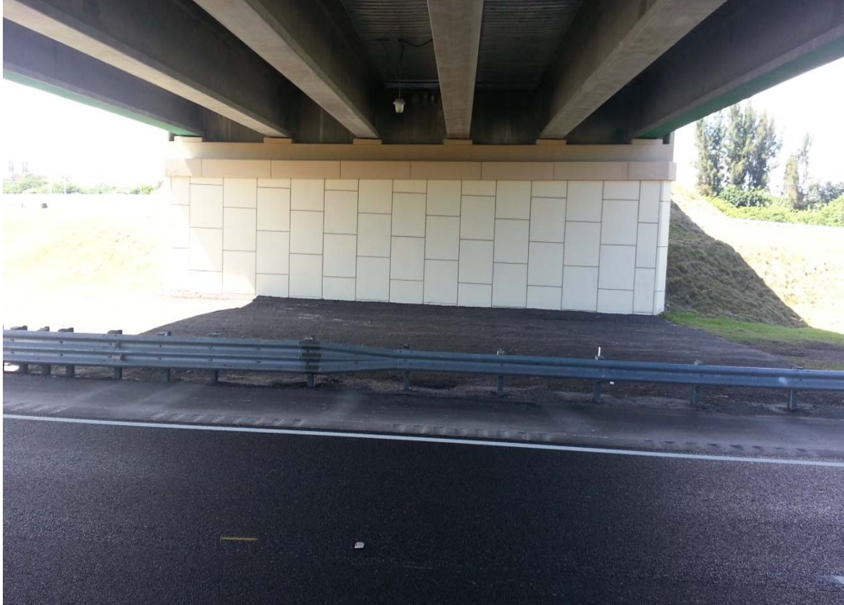
Figure 6 – Millings in Lieu of Performance Turf below Bridge
