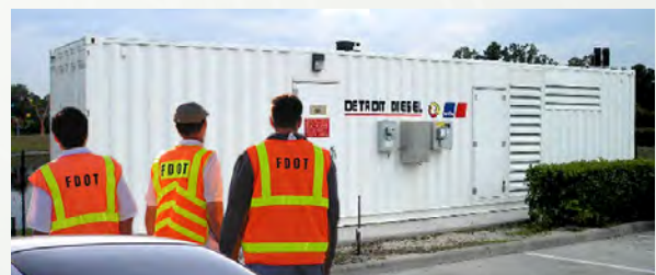
Industrial-size generators provide uninterrupted power for up to 72 hours.
