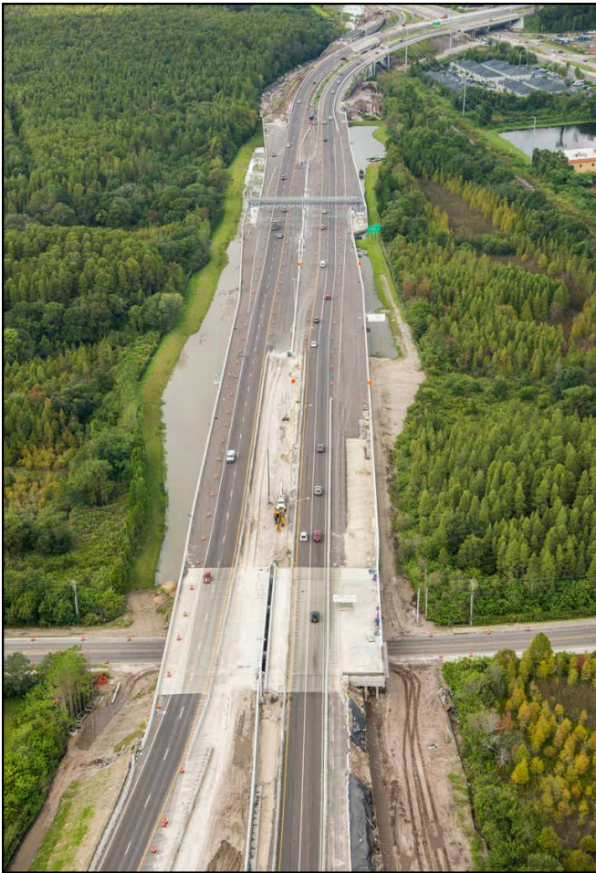
Express lanes on the Veterans Expressway are an integral part of congestion management.
