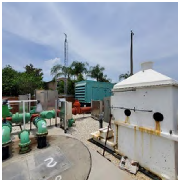
Site 5 – Lift Station 97 North of lift station looking southwest
