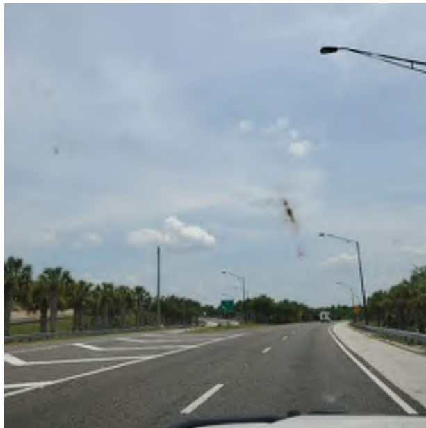
SR 429 Near south project limit looking south
