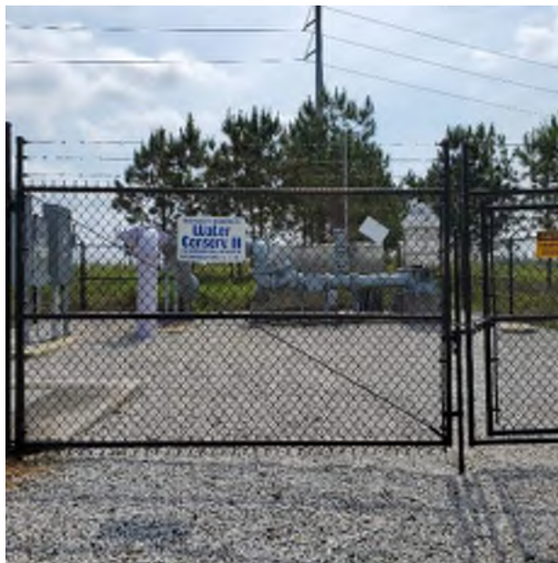
Site 22 – Water Conserve II 3W-01 Supplemental Well West side of facility looking east
