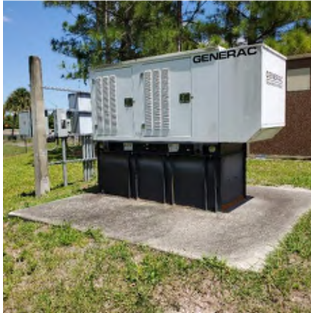
Site 12 – Toll Plaza 5602 Diesel generator with base AST located northwest of Administrative Office
