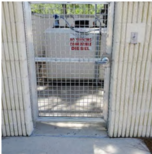
Site 12 – Toll Plaza 5602 1,000-gallon diesel AST located southwest of Administrative Office
