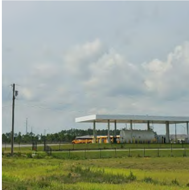
Site 20 – Horizon High School SR 429 looking east at fuel facility with 15,000-gallon diesel AST
