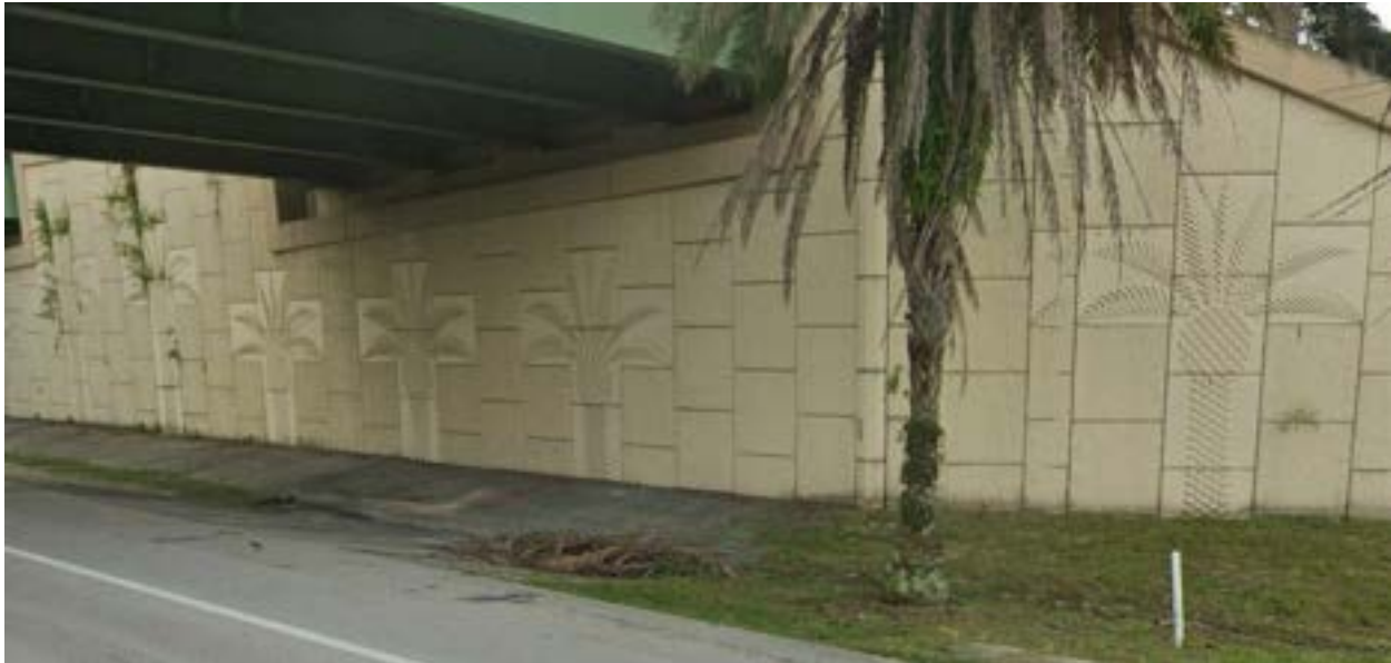
Figure 2-28: MSE Walls at the US 192 Interchange
