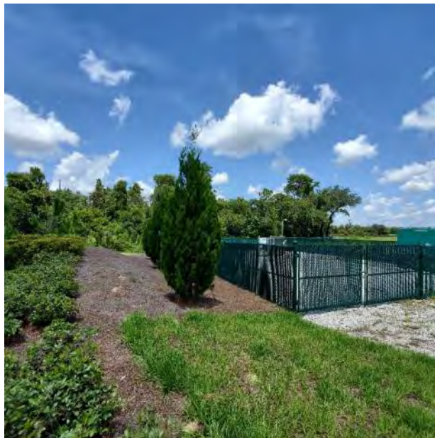
Site 15 – Lift Station Southeast of lift station looking west
