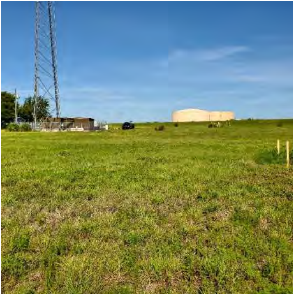
Northeast corner looking west
