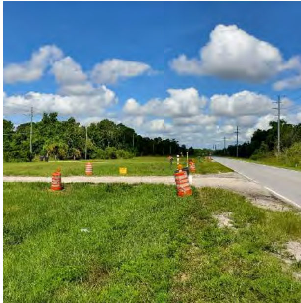
Osceola Polk Line Road (CR 532) looking west Southern portion of project
