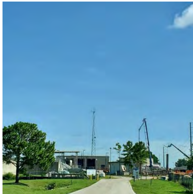
Site 19 – Sand Hill WWTP South entrance of WWTP looking north
