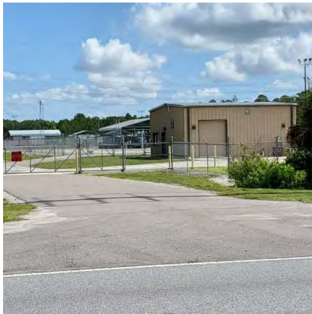
Site 6 – Sabal Trail Transmission Reunion Southwest looking northeast
