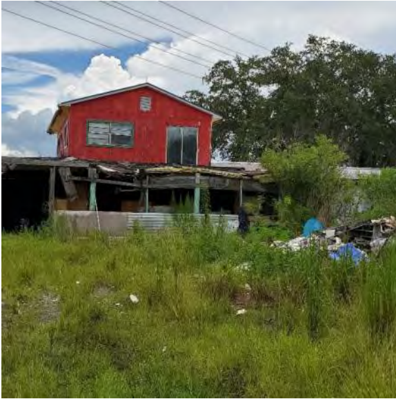
West of structure looking east
