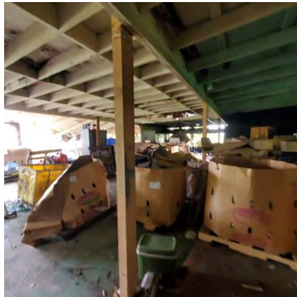
Interior of building
