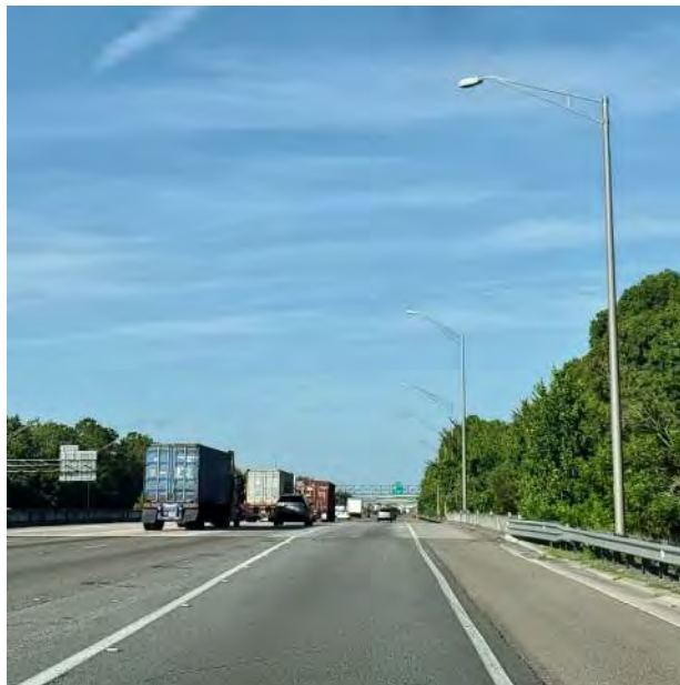
I-4, near east project limit looking west
