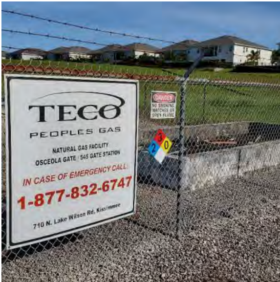
West side of facility looking northwest
