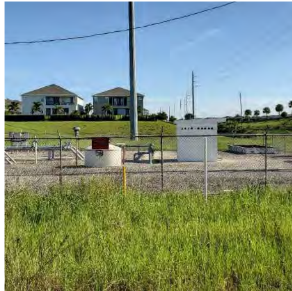
South of facility looking north
