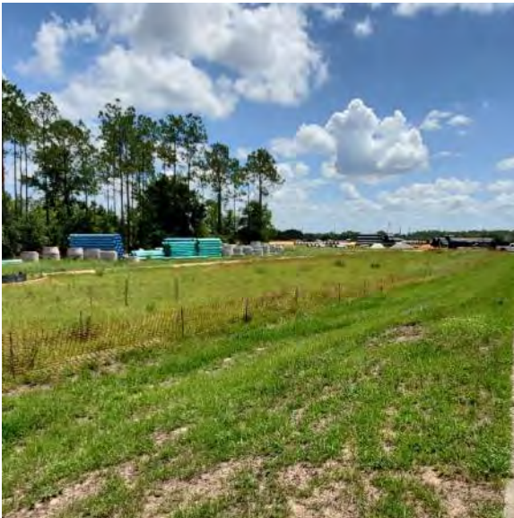
Near south boundary looking northeast
