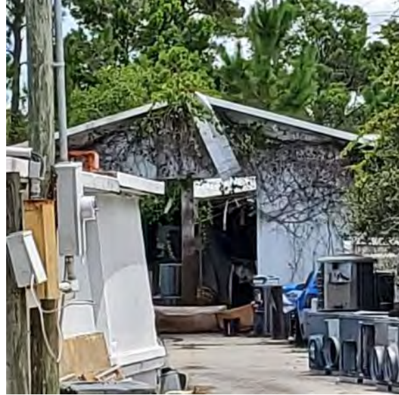
South of storage building looking north
