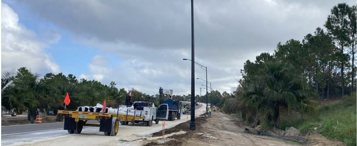
Figure 6: Photo of a ramp on the I-4 and SR 429 interchange showing the existing landscape and the current impacts of construction. Tree protection barriers should be utilized to protect the landscape to remain.
