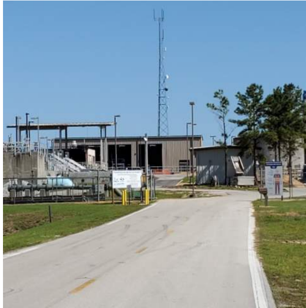
Site 4 – Sand Hill WWTP Southeast corner of WWTP looking north
