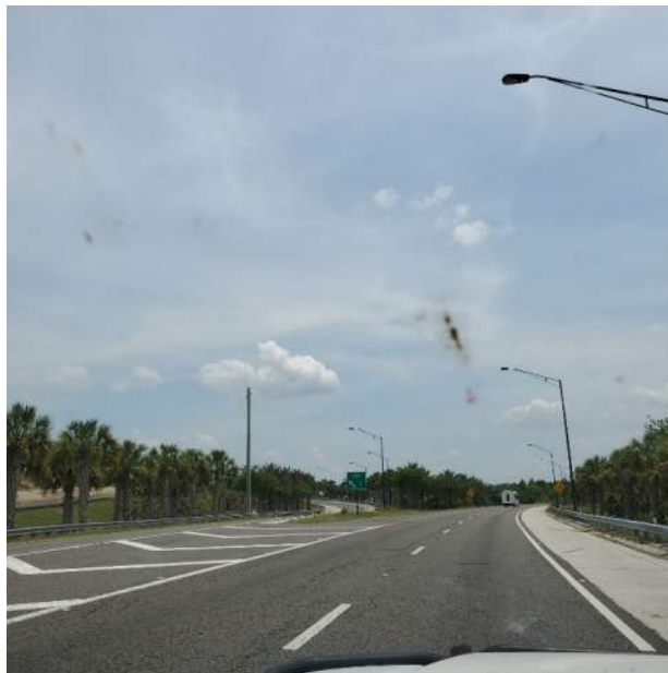
SR 429 Near south project limit looking south
