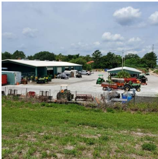
Site 14 – Orange Lake Resort/The Legend Golf Course maintenance facility West of SR 429 looking west
