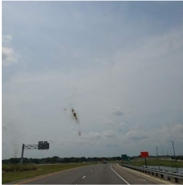
SR 429 Near north limit looking south
