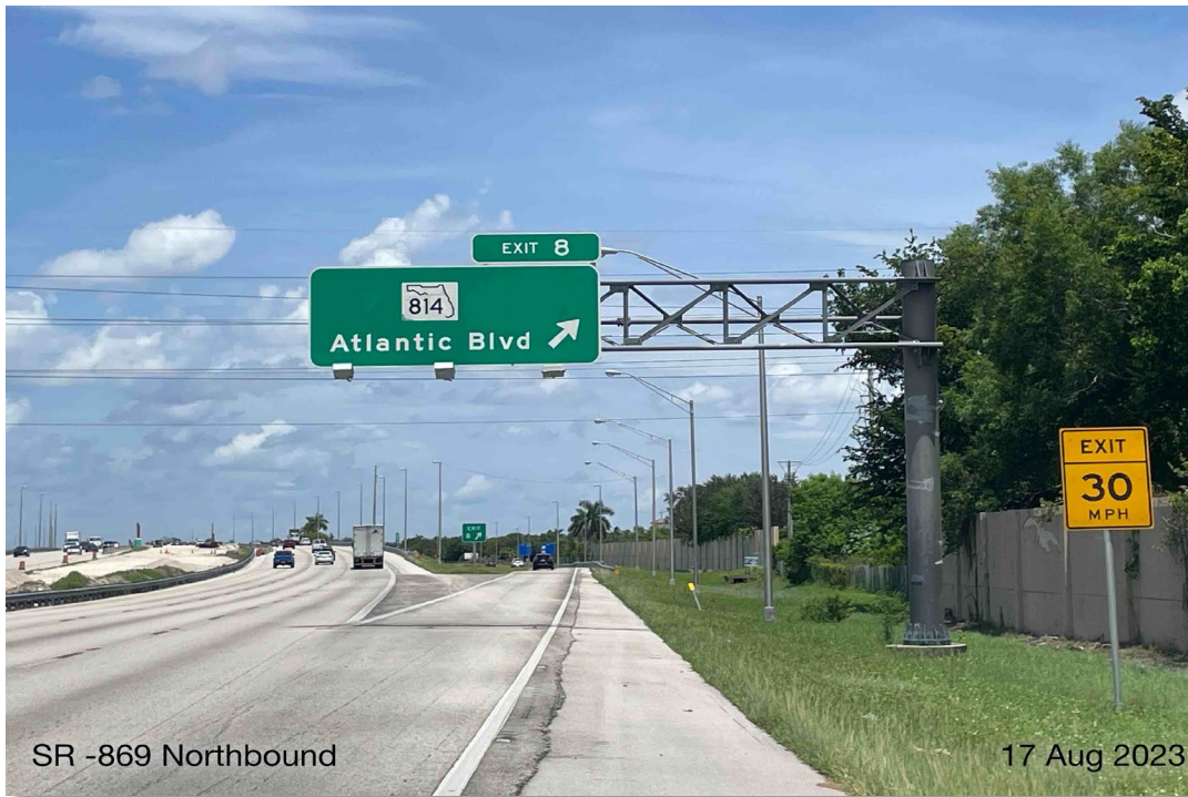
Figure 9: Overhead Sign Structure
