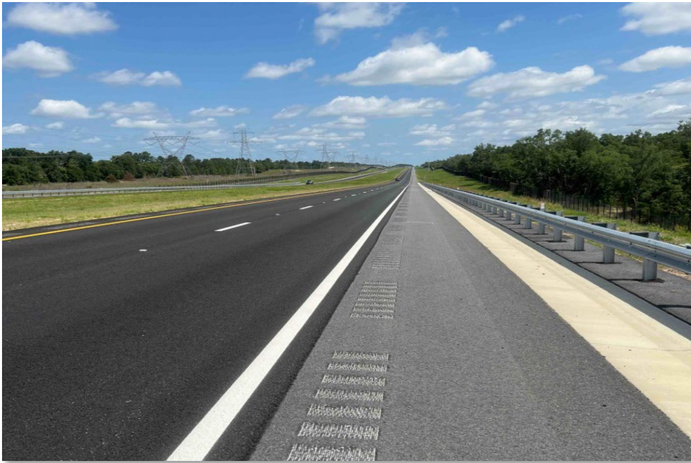
Desired Shoulder Gutter
