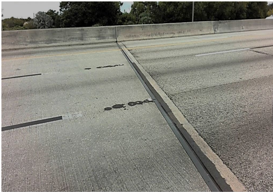
Desired Joint Condition
