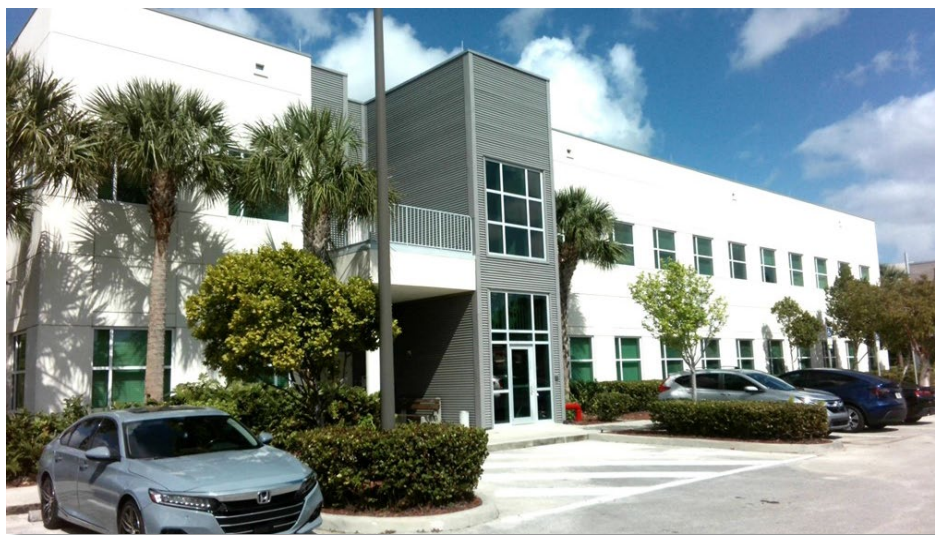
Figure 7: Pompano Operations Annex Building – SR 91
