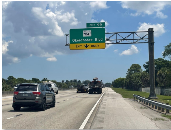
Figure 16: Typical Overhead Sign Structure
