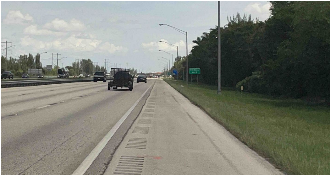
Figure 10: Typical Paved and Soil Shoulder Section
