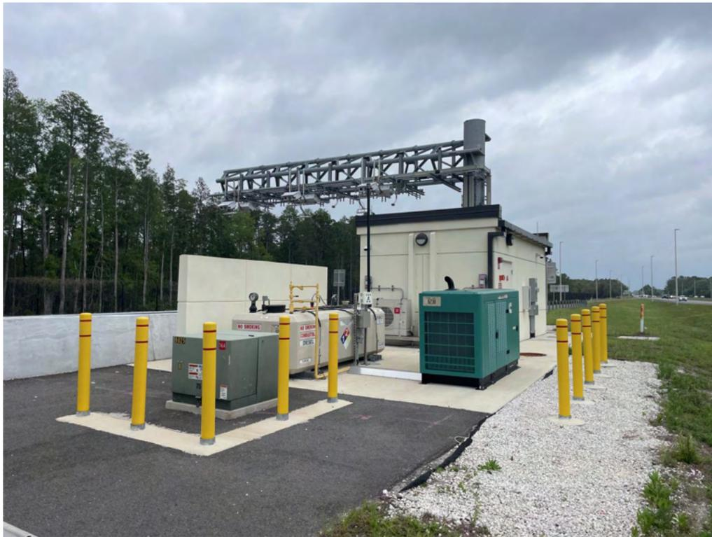
**Site 22 – Toll Gantry at Ridge Road (Suncoast Parkway Interchange at Ridge Road); View of two 500-gallon diesel ASTs located on the northbound on-ramp and southbound off-ramp.**
