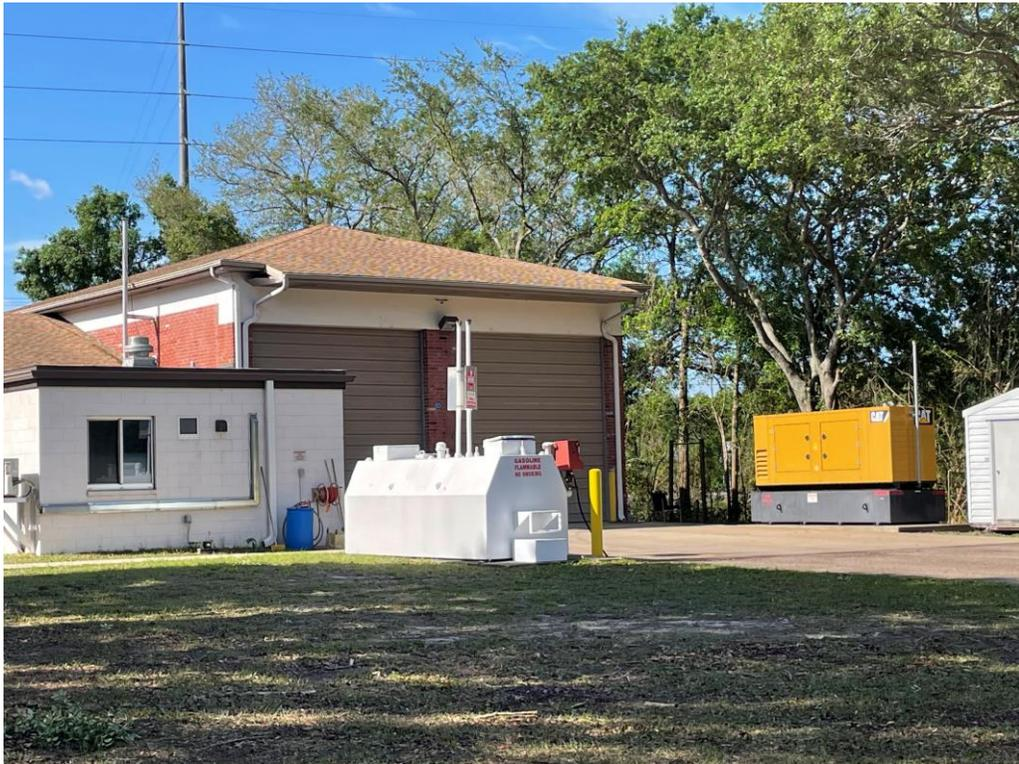
**Site 07 – Hillsborough Cnty Fire Dept #34 (6415 Van Dyke Road); View of 750-gallon emergency generator diesel AST and 1,000-gallon vehicular diesel AST, located off the north side of the fire station building.**
