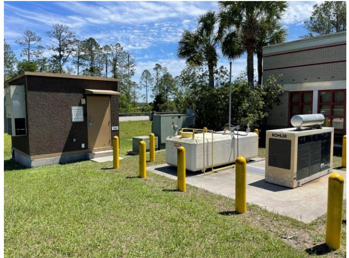
Site 01 – FDOT Florida’s Turnpike Enterprise Anclote Toll PI (6610 Suncoast Pkwy); View showing southern building with 1,000-gallon emergency generator diesel AST; view of 500-gallon emergency generator diesel AST on north side of northern building.
