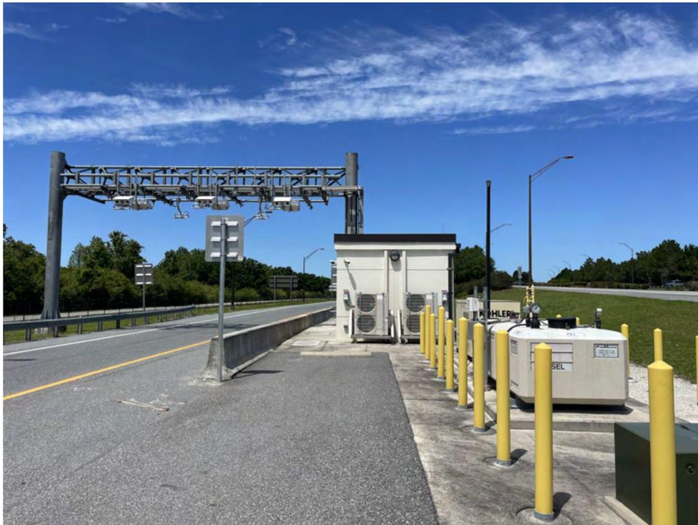
**Site 21 – Toll Gantry at State Road 54 (Suncoast Parkway Interchange at SR 54); View of two 500-gallon diesel ASTs located on the northbound off-ramp and southbound on-ramp.**
